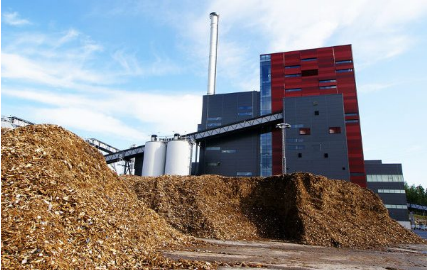
biomassacentrale (foto 123rf)
